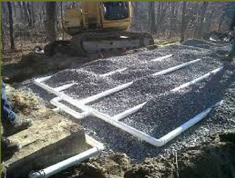
A typical class 4 septic system under construction
